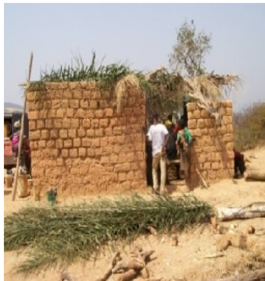
(Mud church construction in Cameroon)
