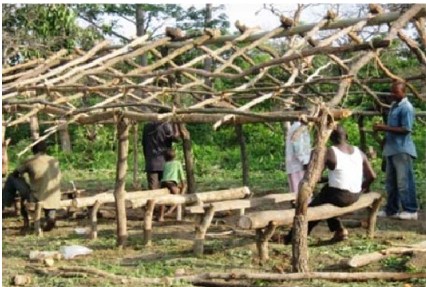
a church under construction
