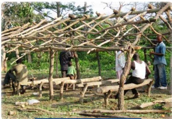
Church under construction
