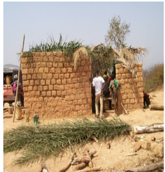
Mud church construction in Cameroon
